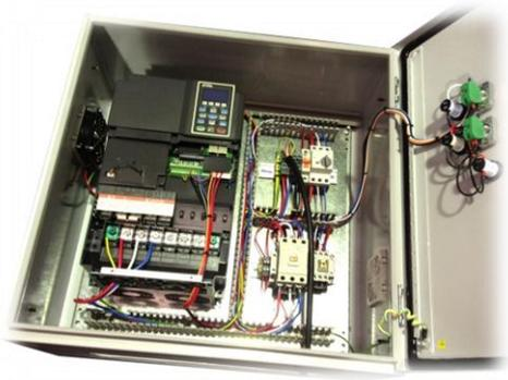
Our **OPTIFLOW** purpose designed Controller automatically controls the fan speed to maintain constant flow in the duct while making very significant savings in electrical consumption.
